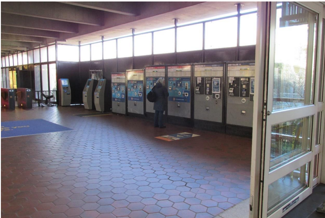
The vestibule of the Metro Station at Reagan Airport. Card-vending machines are there, and electronic turnstiles are beyond the machines.
